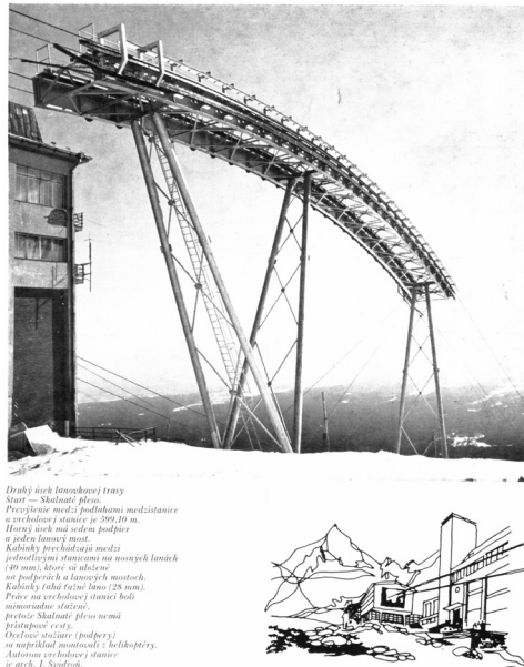
Fig. 5: The inside back cover of the magazine Projekt presents the Skalnaté pleso gondola as a “cutaway”: a photograph of the so-called cable bridge in front of the Skalnaté pleso station and a sketch of the station building as an addition to Dušan Jurkovič’s original station. The new station was designed by the architect Jozef Švidroň (1907–1998). 42
